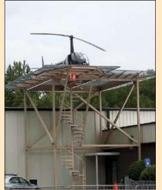
The new Robinson-built helipad is supported by a free standing, 24-foot high steel platform.
