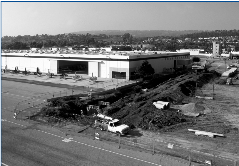
Ground preparation for Robinson's new 215,000 sq. ft. building.
